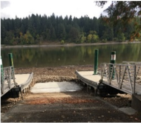
Boat Ramp Repaired!
