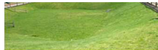
This detention pond is an example of a stormwater facility.
