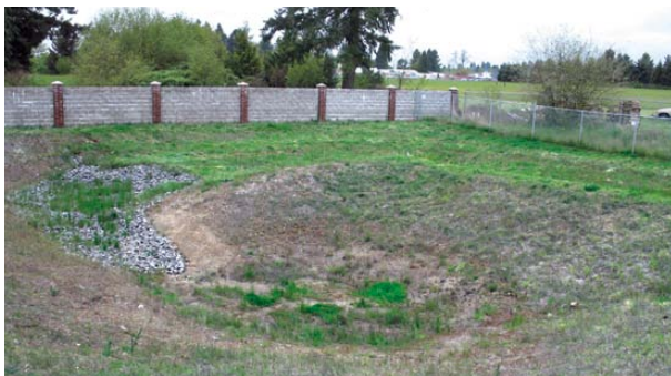
▲ Infiltration basin (page 12) is an open basin that holds water while it soaks into the ground.
