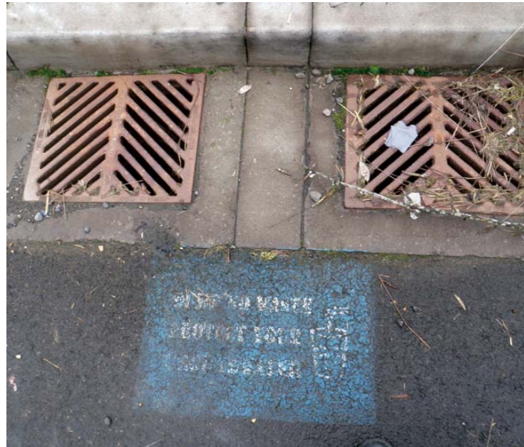
Above: Catch basin (storm drain).
