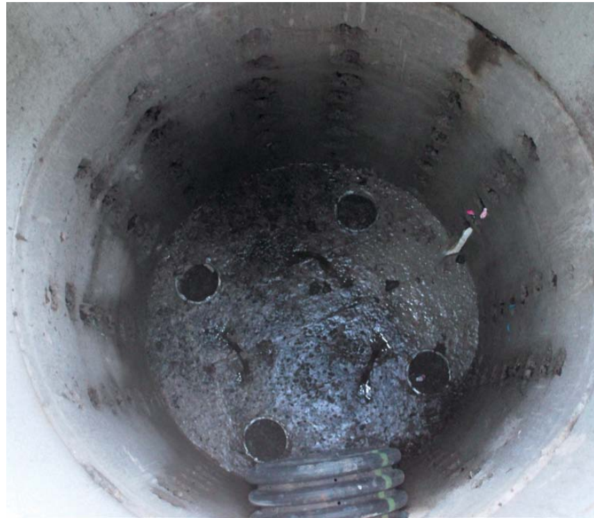
◀ ▲ GOOD: Left photo shows the typical lid of a drywell. Above is a well maintained interior.
