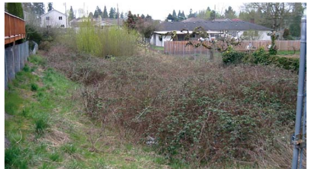
▼ PROBLEM: Noxious weeds have taken over this biofiltration swale.
