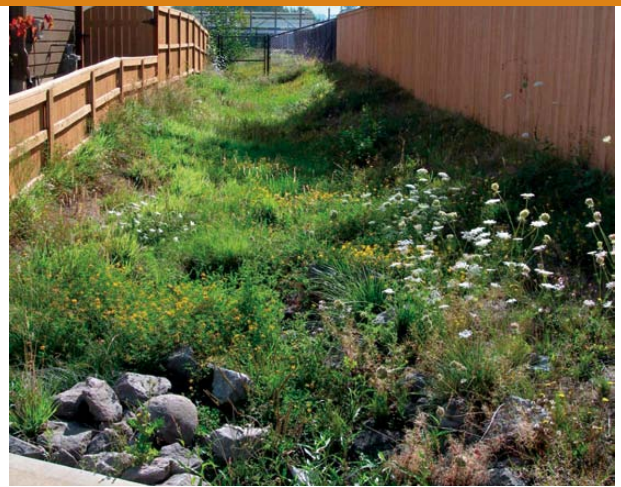
▲ GOOD: Well maintained biofiltration swale.
