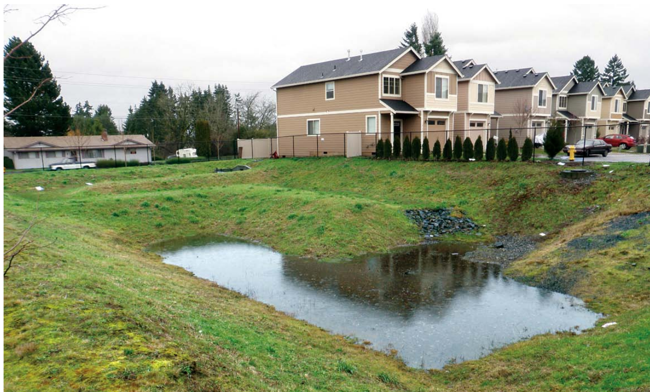
GOOD: Above shows a dry infiltration basin. Unlike a detention pond, an infiltration basin has an underground structure that helps water soak into the ground. Below is a good basin shortly after a rain storm.
