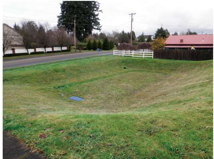
GOOD: Above shows a dry infiltration basin. Unlike a detention pond, an infiltration basin has an underground structure that helps water soak into the ground. Below is a good basin shortly after a rain storm.
