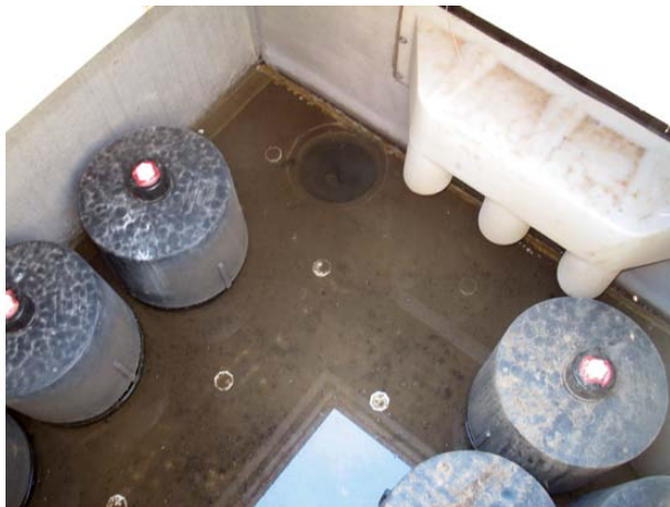
GOOD: Well maintained interior of a stormwater filter vault facility.
