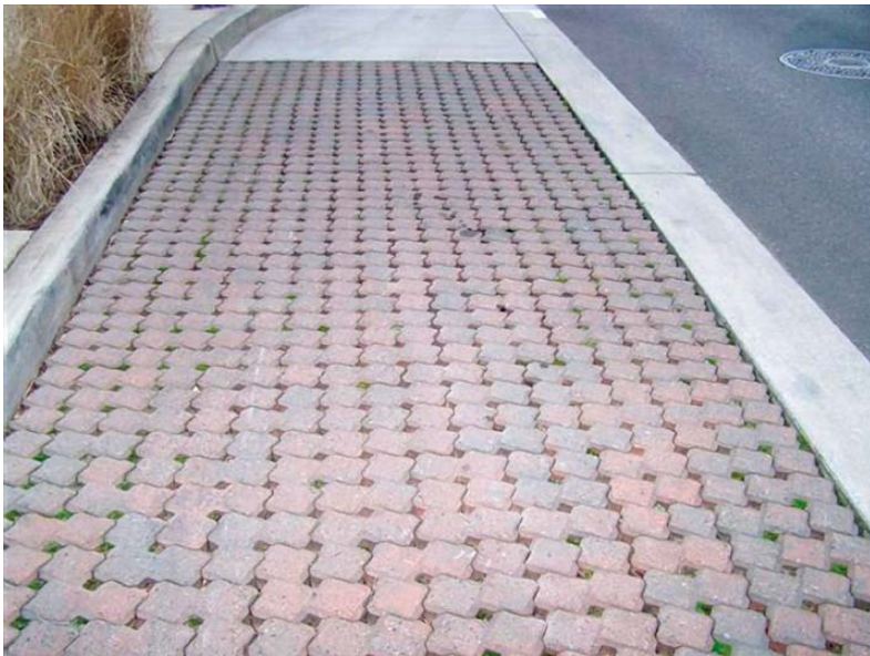
Pervious pavers, note the spaces between the pavers.
