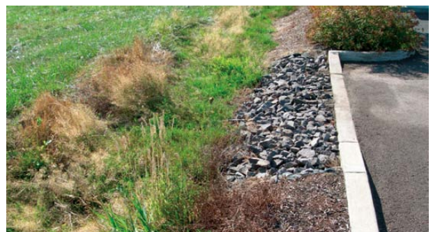
▼ Filter strip (page 9) is a strip of grass along paved areas such as a road or parking lot. Contaminants are filtered out of the water as it flows away.
