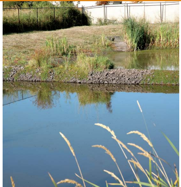
GOOD: Well maintained examples of wetponds. Above shows a two-pool wetpond.
