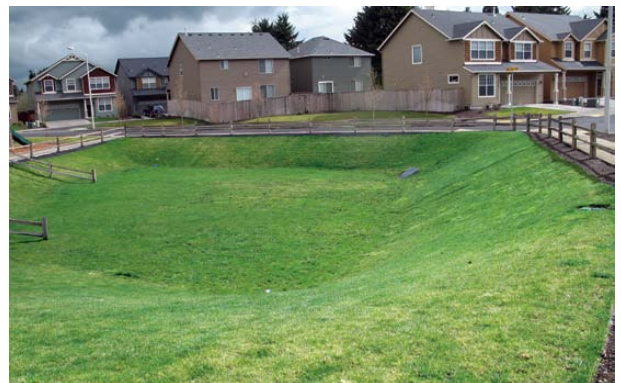
▲ Detention pond (page 11) Stormwater is temporarily stored and slowly released through an outlet pipe. Natural-appearing vegetation is common.
