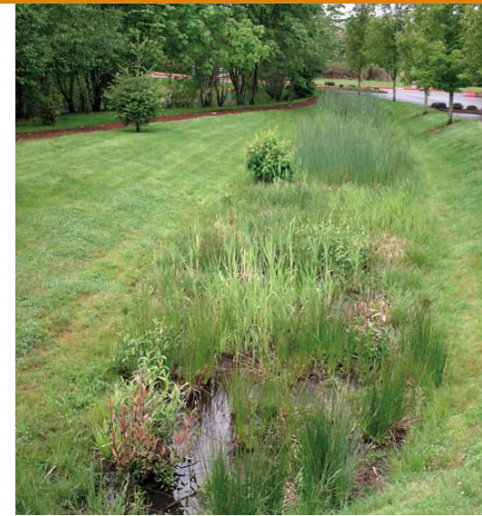
GOOD: Both photos show well maintained detention ponds. Shortly after a rain storm, the pool of water, above, is slowly draining. On the left, the pond is dry between storms.
