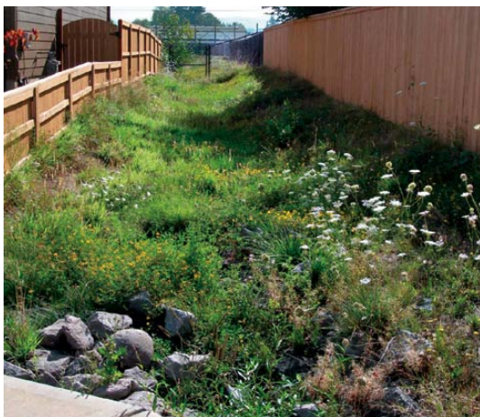
▼ Biofiltration swale (page 9) is a flat-bottomed channel where pollutants are removed by filtration, infiltration and settling.
