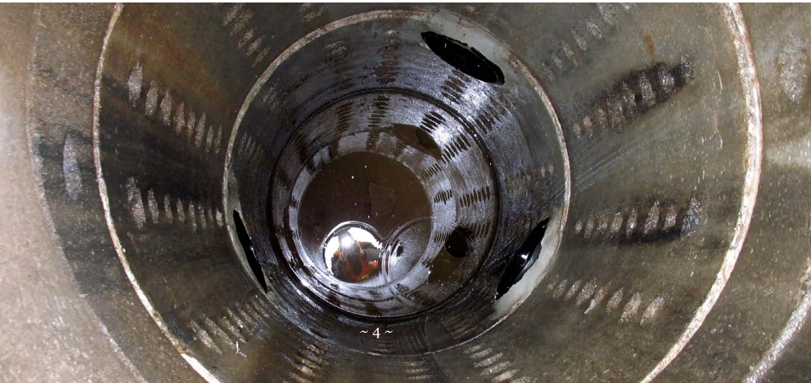
A well-maintained drywell has no debris or standing water. This photo shows water draining after a rain storm. The holes around the wall allow water to soak into the ground. See page 18 for more information about drywells.
