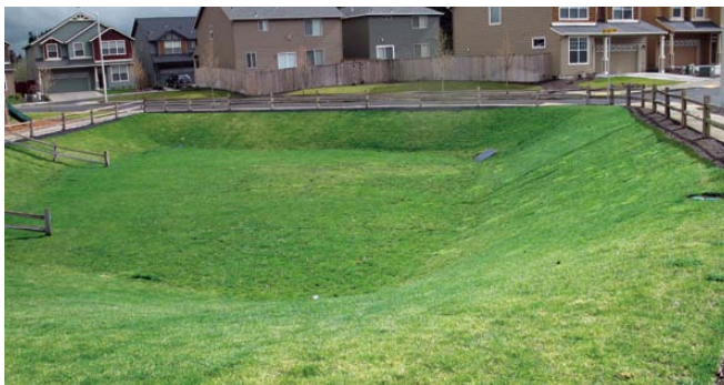
GOOD: Both photos show well maintained detention ponds. Shortly after a rain storm, the pool of water, above, is slowly draining. On the left, the pond is dry between storms.
