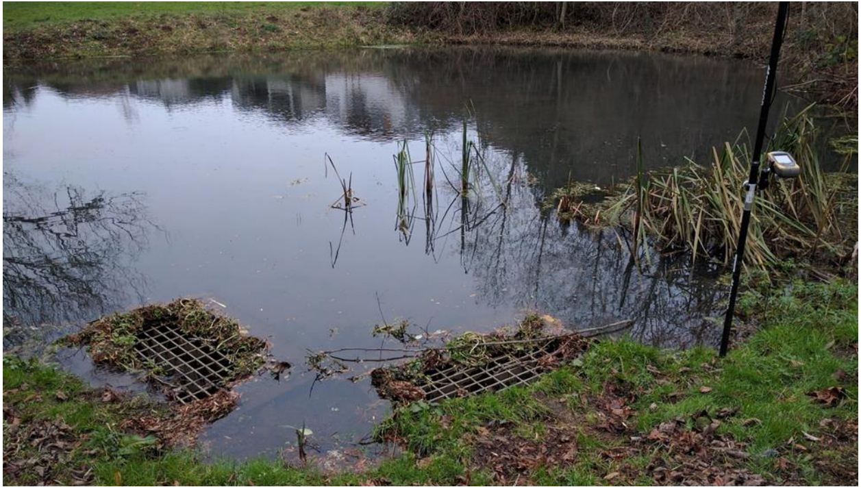
Photo 3. Settling pond and drains built as part of the 1996 Stormwater modification.
