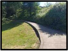
This line item "Step Replacement & Restabilization" has been removed (and unfunded) from this reserve study as the wooden railroad ties have been since replaced with a concrete pathway. This line item is a placeholder and serves notification to the reader that the line item has been removed from this reserve study.
